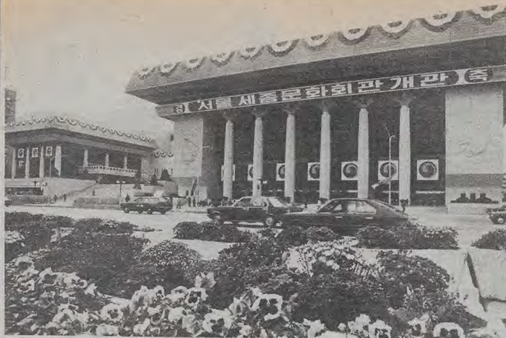
This is the front view of the Seoul Sejong Cultural Center in Kwanghwamun. The impressive complex was dedicated yesterday.
